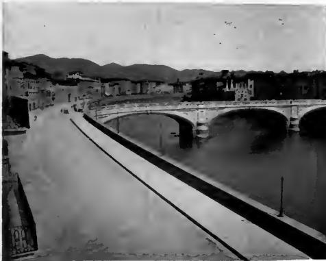
Embankment of the Arno at Pisa.
